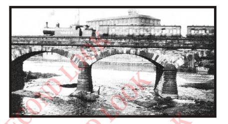
Lancashire & Yorkshire Railway 2-4-2 passing over Newgate bridge. The bridge in the present view was built alongside the original stone viaduct in 1930 when the number of tracks were increased to two up and two down workings.
