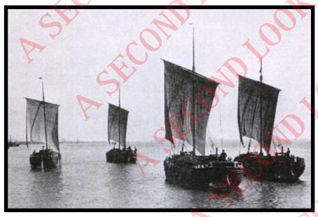
West country boats were built to a maximum length of 57ft 6in and breadth of 14ft 2in this being the maximum size able to pass through the locks of the upper Calder and Hebble Navigation, although smaller than their Humber cousins they were still capable of sailing onto the tidal estuaries of the Humber and were the only barges capable of crossing the country fully from coast to coast.
