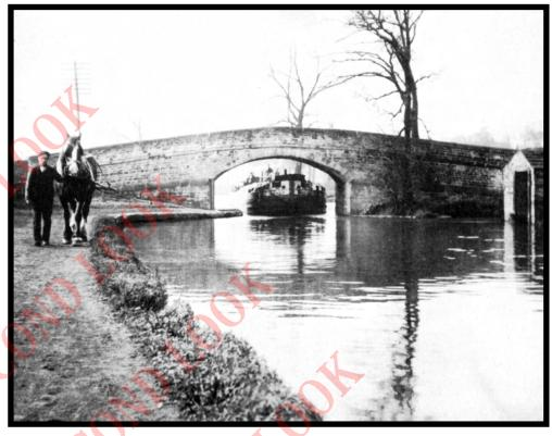
Although West Country Keels were capable of sail this was largely reserved for the Humber and larger sections of river. As seen on the canal at Shepley bridge above the horse was the more common method of power.
